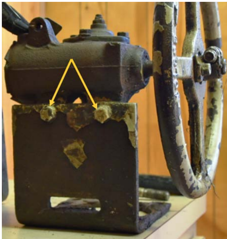
Figure 6. Gearbox support bracket for the valve involved in the incident. The two horizontal bolts (yellow arrows) can be removed to take the gearbox off the support bracket and the valve without disturbing the top-cap bolts. By removing the gearbox in this manner, the pressure-retaining valve components are not disturbed.
